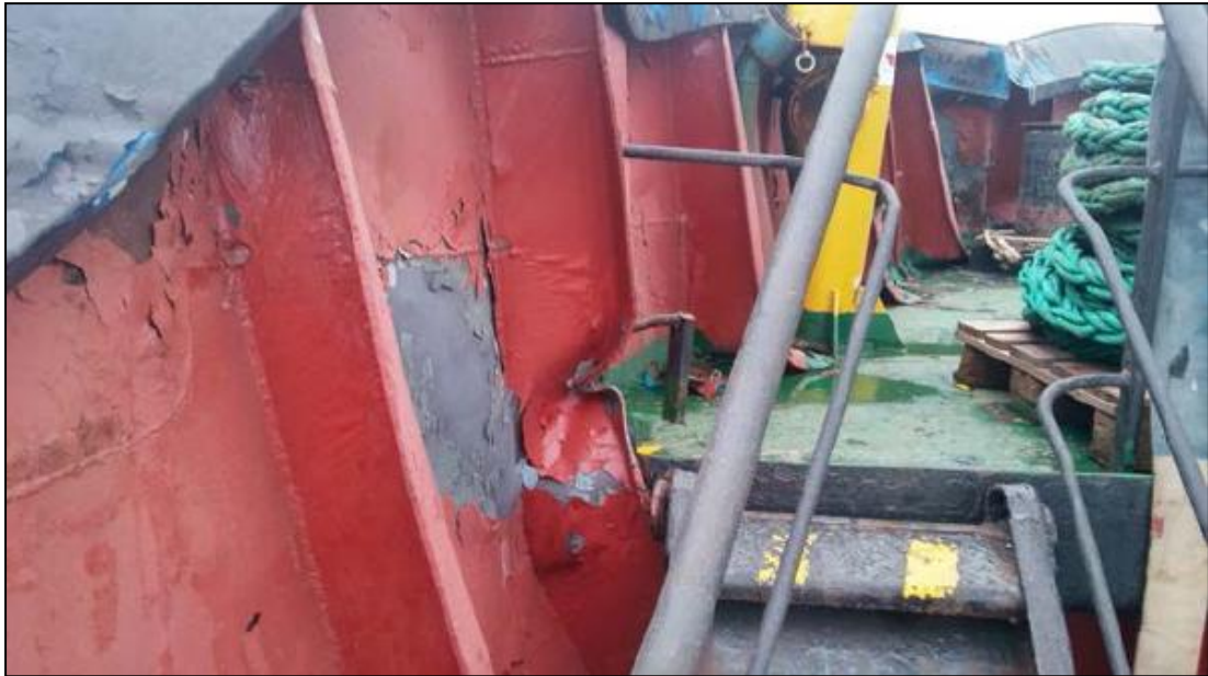
Figure 13: Damages to the forecastle deck
