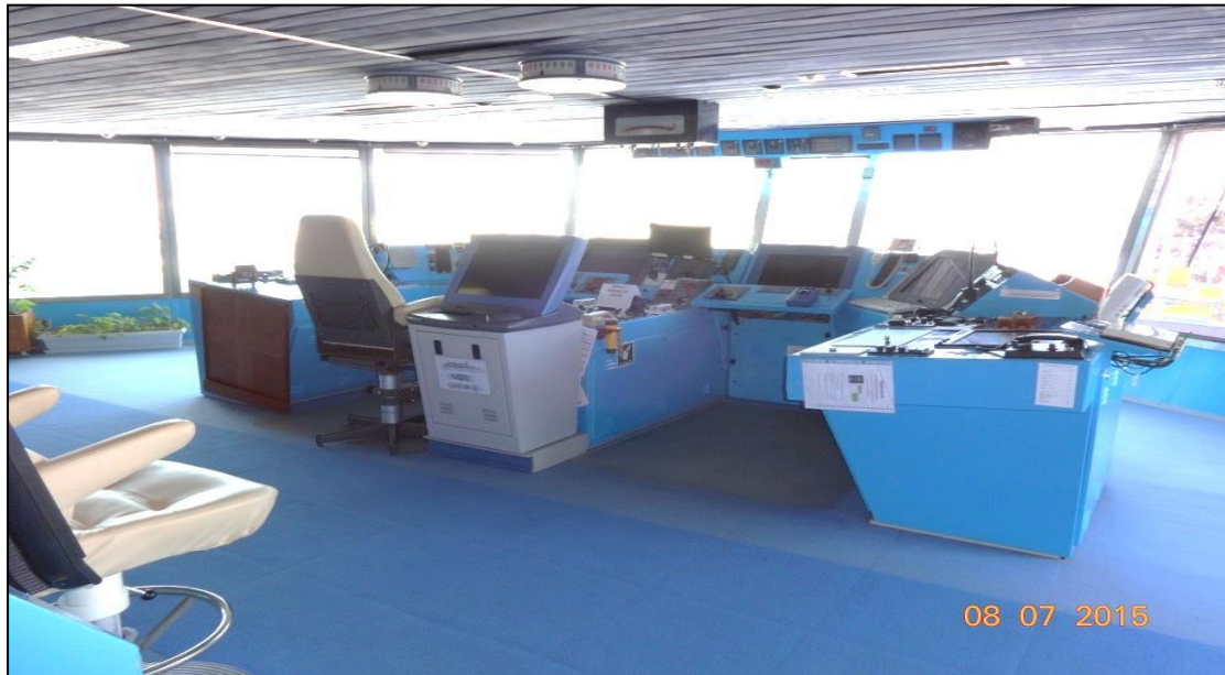
Figure 3: Main bridge console
