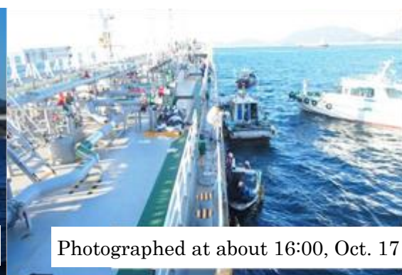
Photo 2.9-2 Oil Recovery Work with Oil Absorbing Mats
